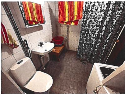
As 1 pesuhuone saneerattu.
